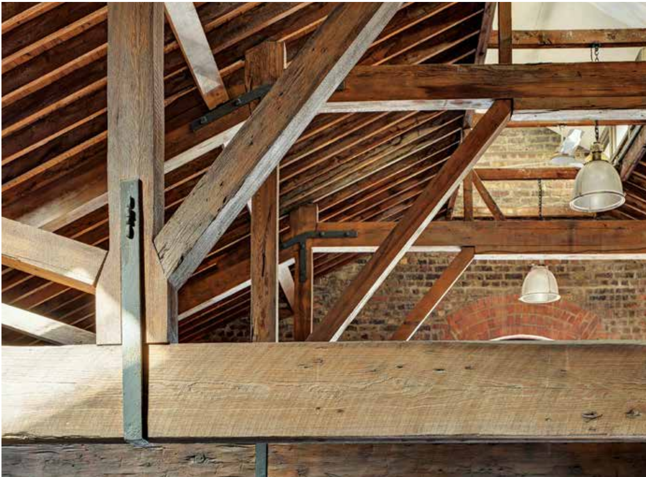
Pictured above Original timber beams at Tropical Fruit Warehouse, Sir John Rogerson’s Quay, Dublin 2
