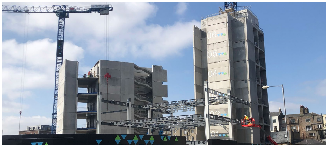
Pictured: One Wilton Park, Dublin 2, under construction
