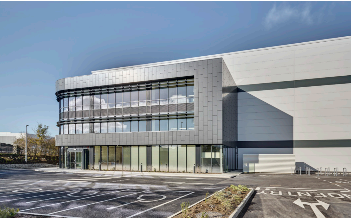
Aerodrome Business Park, Co. Dublin
