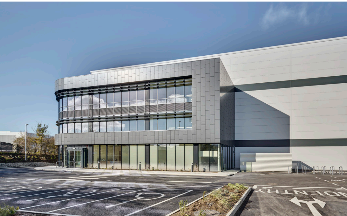
Aerodrome Business Park, Co. Dublin
