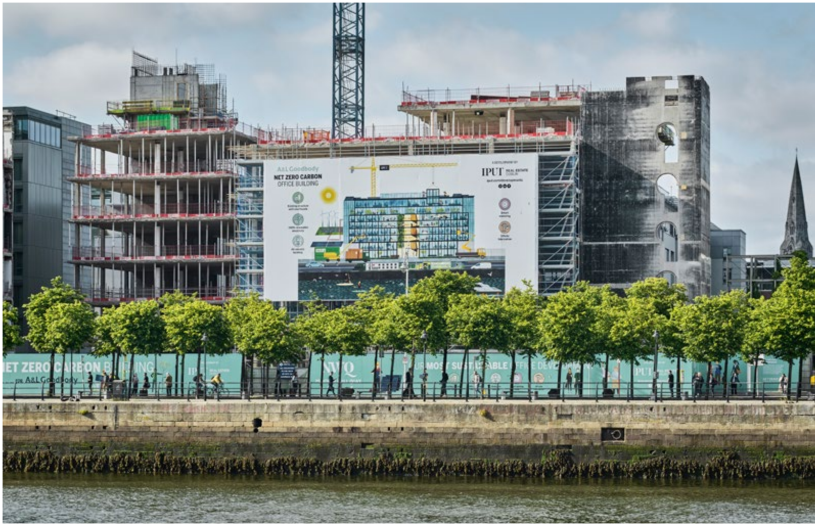
Construction works at 25 North Wall Quay, Dublin 1.
