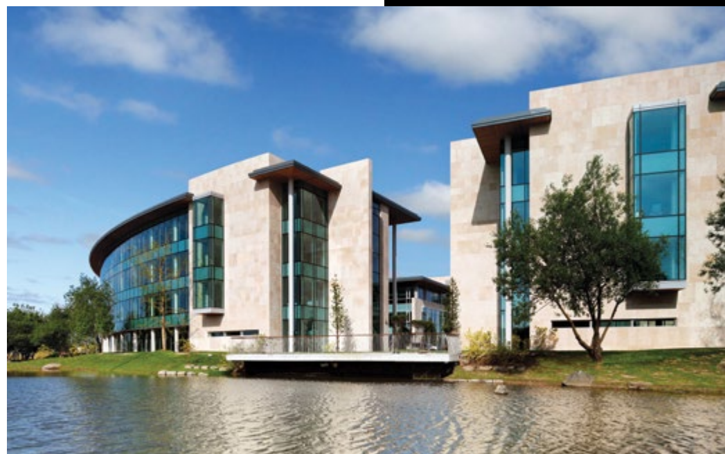
Waterside, Citywest Business Campus, Dublin 24.
